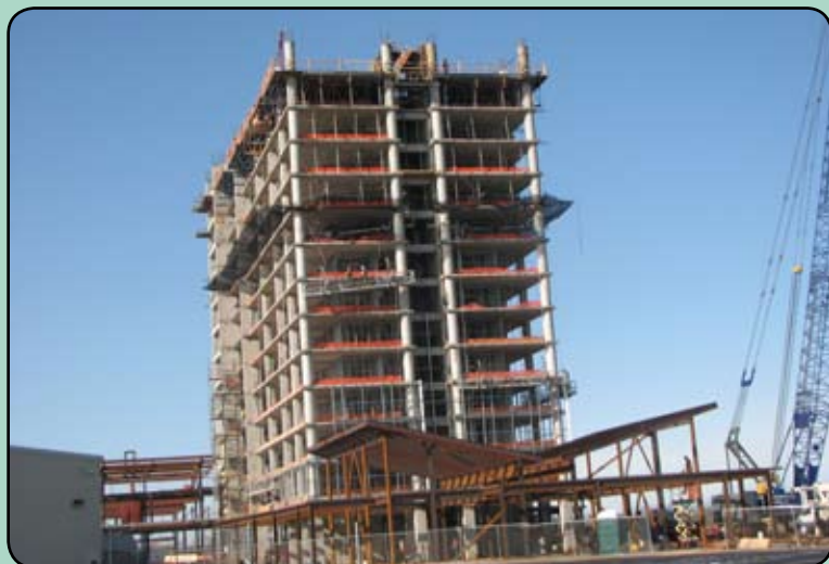
Hotel Tower with 15 th Floor in Place
